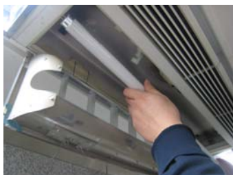
Retirar as lâmpadas tubulares T8
