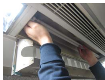
Instalar as lâmpadas tubulares T5 com balastro electrónico
